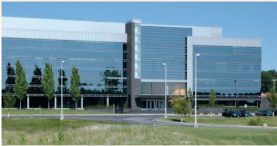
NDI Medical Headquarters in Cleveland, Ohio
